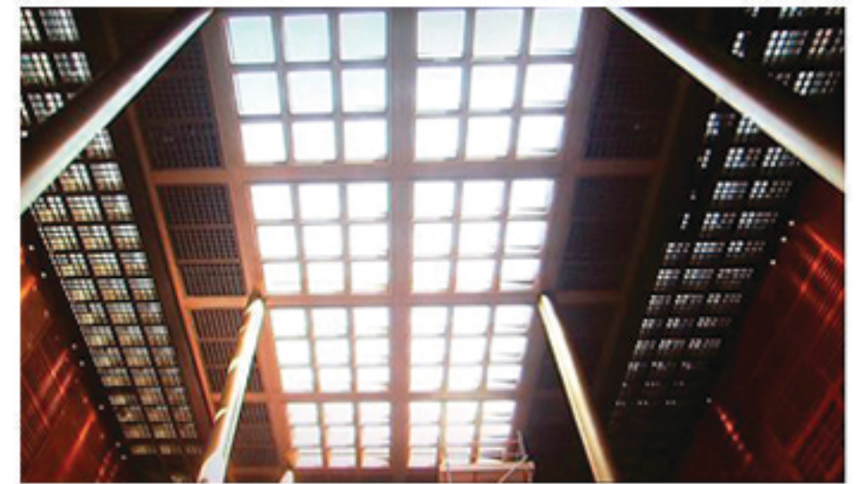
3. Roof system fully open, allowing sunlight to penetrate brightening interior spaces. Each unit is driven by a servo motor with custom array control.
