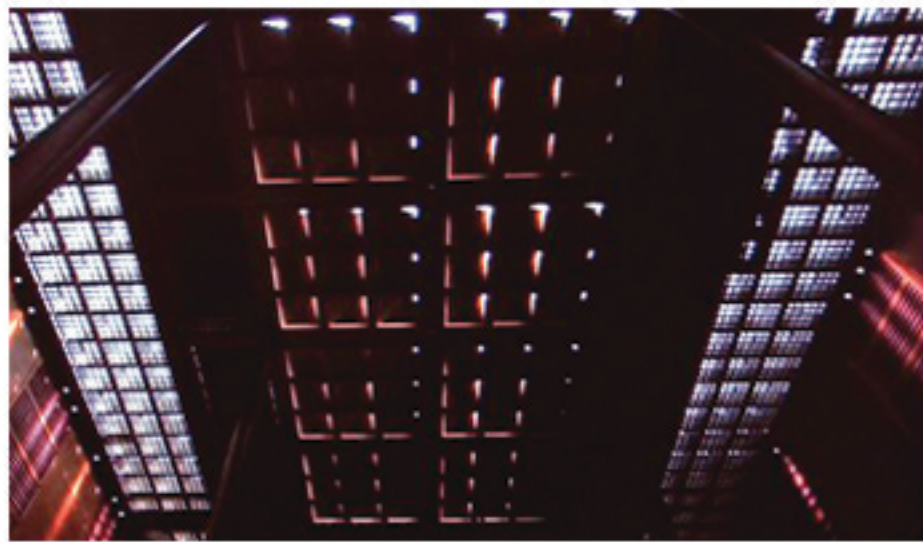
1. Roof system closed. Panels fully stretched out, shading interior spaces.
