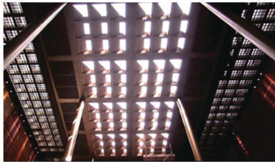
2. Roof system start to interact. The panels move parallel to the building's surface, allowing its layers to be completely hidden when retracted.
