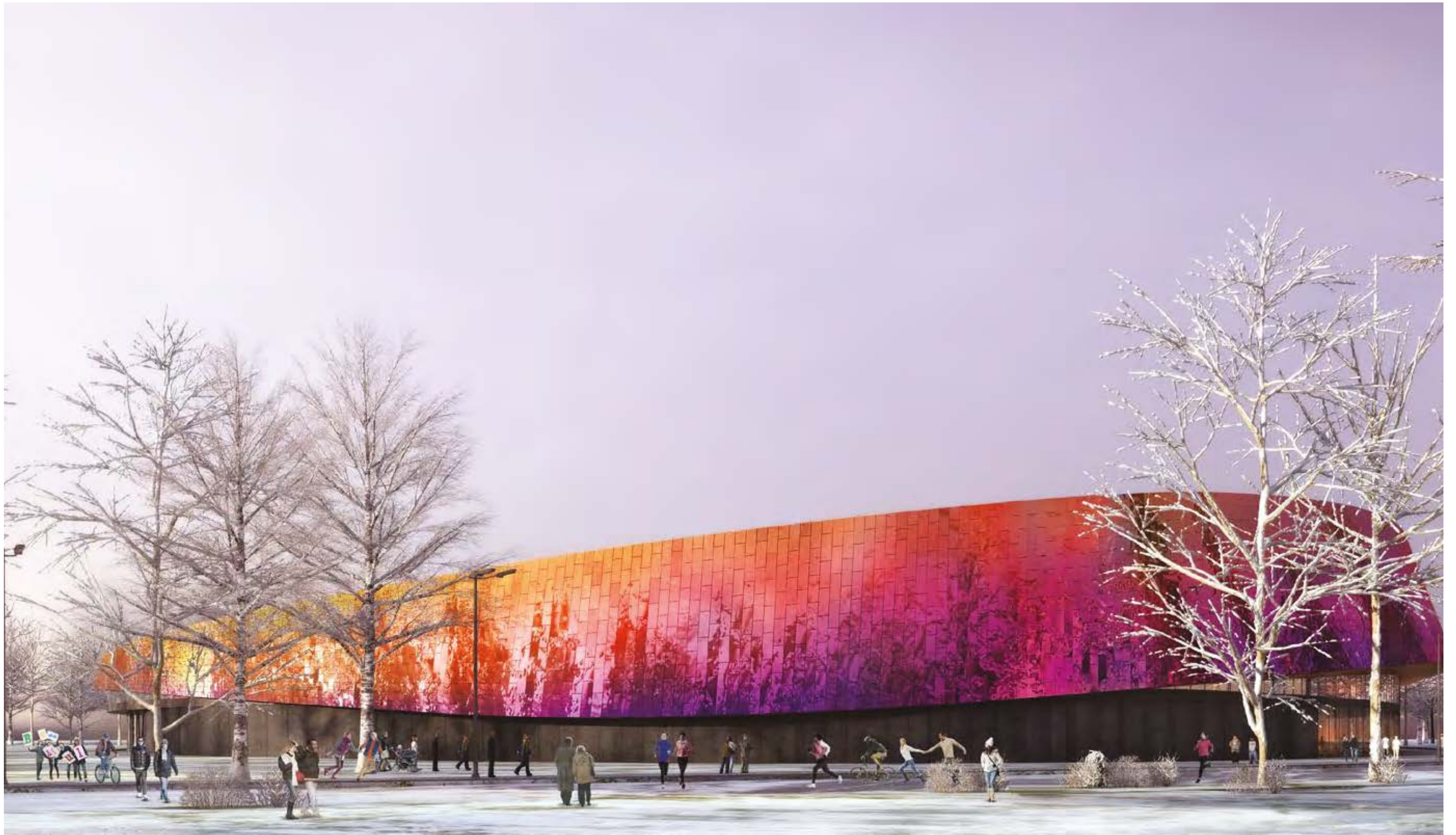
SPORTCAMPUS ZUIDERPARK - ABT (CONSULTING ENGINEER)
